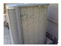
Condenser coil (Outdoor coil) that is not maintained can cause part failure and inefficient operation.
