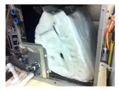
Dirty Filters and restricted air flow can lead to freezing. This can lead to water damage in your home and failure of many components.
