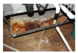
Improper drainage can cause your drain pan to rust and that can lead to future water damage.
