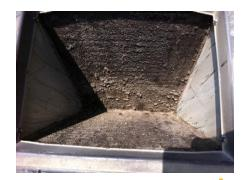
Evaporator Coil (Indoor coil) because of dirty filters. This can lead to major service issues and home damage.
